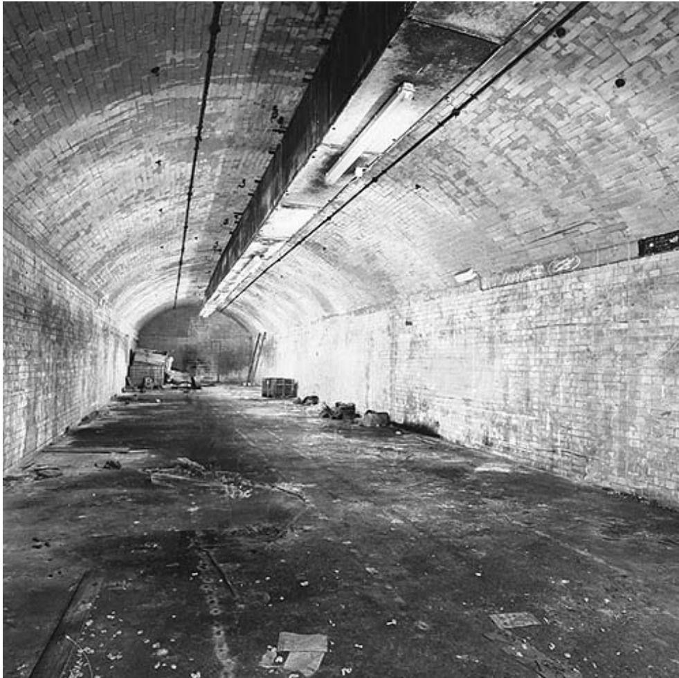
Shorts Brothers - One of the 100 metre factory tunnels
